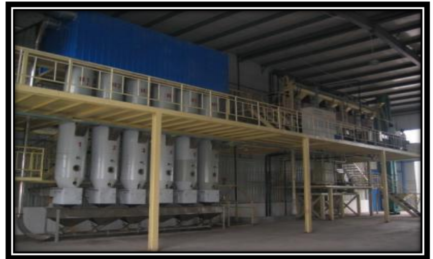
Sesame Peeling & Follow-Up Processing Section After installation I
