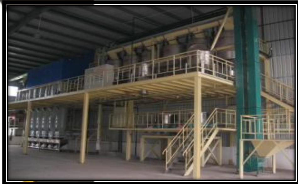
After Installation II
